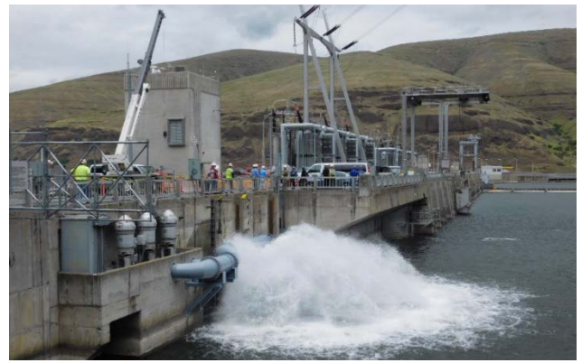
Water cooling systems were installed at Lower Granite and Little Goose dams in 2016 and 2017.
